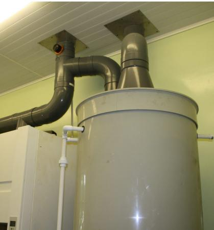
The scrubber is designed for recovery acids vapor in the air flow coming out of exhaust hoods in laboratories.
